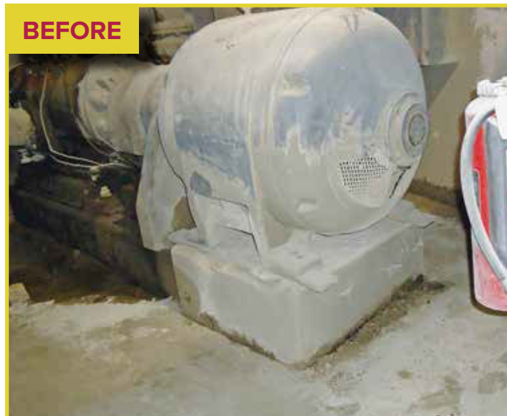
On-site turnkey retrofit of a new 500 HP pump motor, base design, fabrication, and installation.
